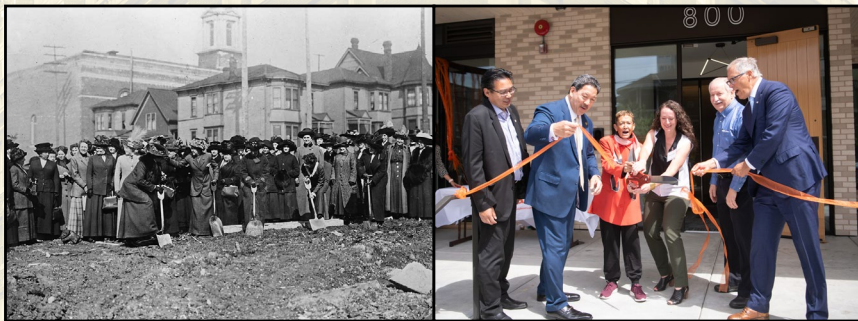
Breaking ground at YWCA Seneca, 1913 | Ribbon cutting at YWCA Denny Apartments, 2023
